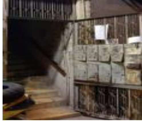
閘門打開，不論住客與否，都可隨便出入，大廈安全成疑 The gate is opened so that someone can pass through it, whether or not they are residents, leading to security problem.
